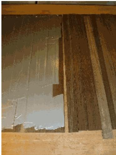
The strips are placed bevel-down on a flat surface, and taped edge to edge with the edges aligned square. Duct tape is excellent, as any viewer of the Red Green show will tell you. To glue the tube strips together, flip them over and squeeze a thin bead of glue into each bevel. Then bend it into a tube shape, and put tape on the last seam.
